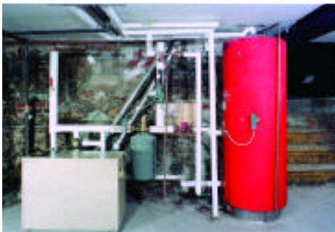
**Indirect water heater shown connected to sealed combustion boiler.**
